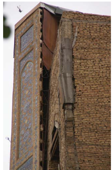
Fig. 15 (right). View of the back section of the iwan screen of the Bibi Khanum, showing separation between it and the reinforced concrete of the towers, 2013.
