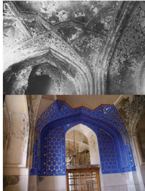
Fig. 35a, b. The Ishrat Khaneh under reconstruction, 2013, where the contrast with Pugachenkova's photo from 1963 demonstrates how much of the interior decoration is being created de novo.
