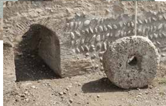
At SHUSTAR (top four pictures), a Sasanian era dam diverted water from the river to a canal that led to town, where horizontal wheel mills (their workings shown in the diagram), lined each side of the waterway. At DEZFUL, vertical wheel mills were built out into a rapidly flowing section of the river, a reconstruction and one of the huge millstones shown on the right.
