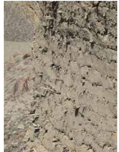
Fig. 4 (right). Detail of the southern wall of Kansir fort, showing brushwood layers between mud-covered bricks.
