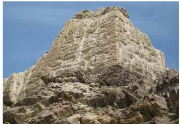
Fig. 5. The southwestern tower of Kansir, showing the stone plinth with mud bricks above.
