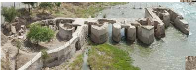
At SHUSTAR (top four pictures), a Sasanian era dam diverted water from the river to a canal that led to town, where horizontal wheel mills (their workings shown in the diagram), lined each side of the waterway. At DEZFUL, vertical wheel mills were built out into a rapidly flowing section of the river, a reconstruction and one of the huge millstones shown on the right.
