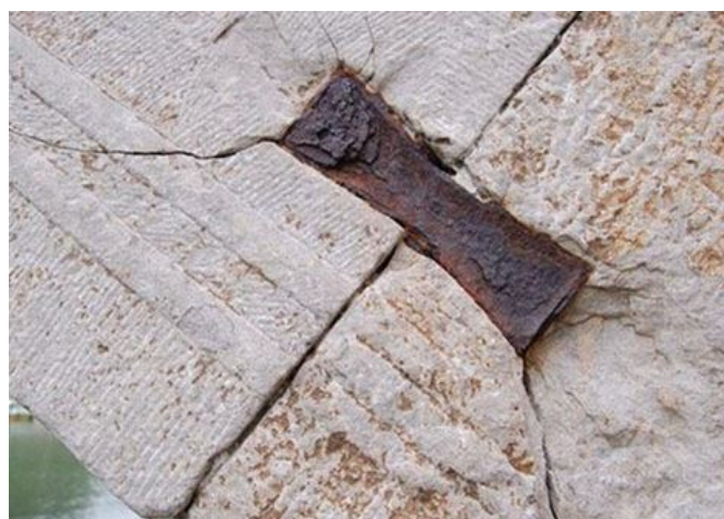
Fig. 9. Top: Zhaozhou Bridge, ca. 600, Sui era, Zhao County, Hebei; Bottom left: Details of dovetail-type clamps (head of the iron tie-bar is circled, while an arrow points to a stone-rivet); Bottom-right: close-up of metal joint clamp.
