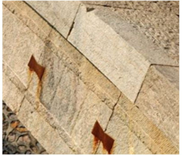
Fig. 10. Left: Yongtong Bridge (open-spandrel segmental arch bridge), ca. 7-8th c., Zhao County, Hebei; Right: details of dovetail-type iron clamps.
