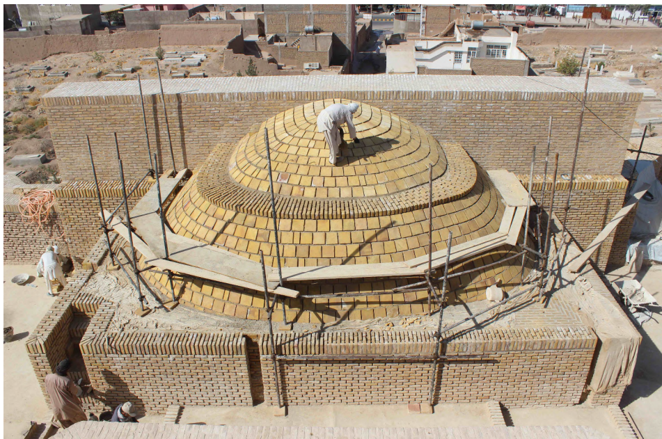
Fig. 11. Brick paving over reconstructed west iwān.
