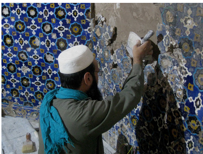
Fig. 19. Pouring gypsum plaster behind unstable mosaic faience.
