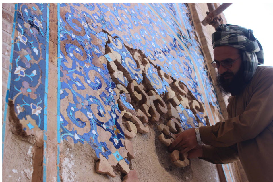
Fig. 12. Conservation of tilework on west elevation.
