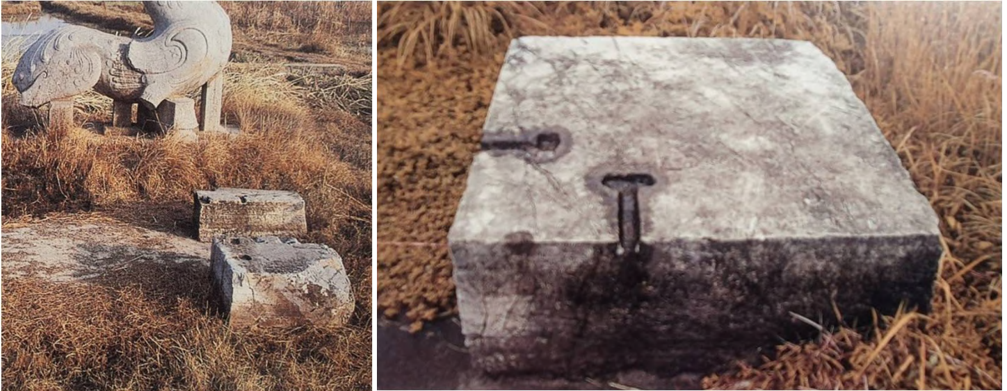
Fig. 12. Left: Stone-blocks with dumbbell-type clamps with circular (or square) heads, Jianling mausoleum of Emperor Wen, Liang dynasty, early 6th c., Danyang (near Nanjing), Jiangsu; Right: A sample block.
