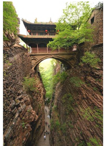
Fig. 11. Above: Qiaolou Dian stone bridge, ca. 7th c. at Xuankongsi Temple, Mount Cangyan, Shijiazhuang, Hebei; Below: Dovetail-type clamps along the span of the segmental arch. (Haphazard repairs impaired the bridge, particularly two spandrels).
