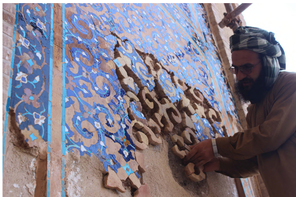
Fig. 12. Conservation of tilework on west elevation.
