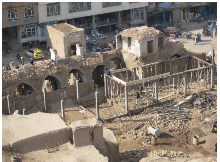
Fig. 24. Demolition of historic property in the old city.
