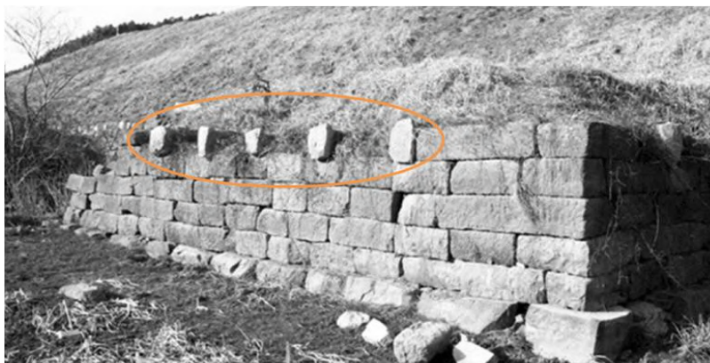
Fig. 14c. Stone rivets on the retaining wall.
