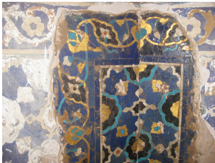
Fig. 20. Mosaic faience concealed behind plaster.
