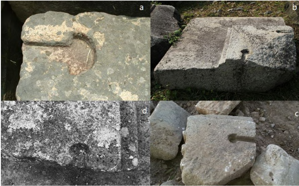
Fig. 17. Examples of half-circle head type clamp grooves from: a) Janghuang-ri temple site, b) Inyong-sa temple site, c) Guhuang-dong temple site; d) Howon-sa temple site. All are datable to latter half of 8th c., Gyeongju.
