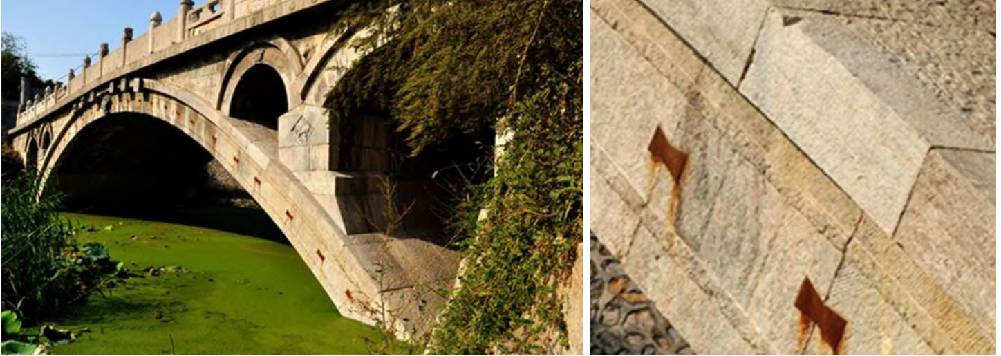
Fig. 10. Left: Yongtong Bridge (open-spandrel segmental arch bridge), ca. 7-8th c., Zhao County, Hebei; Right: details of dovetail-type iron clamps.
