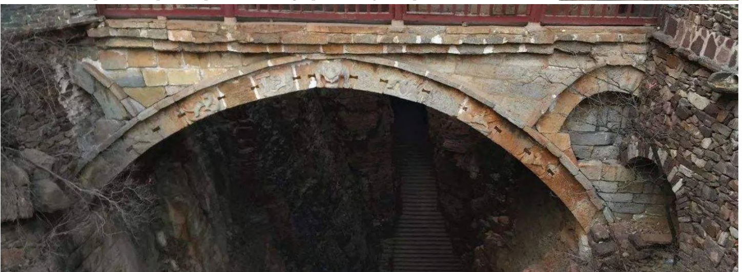
Fig. 11. Above: Qiaolou Dian stone bridge, ca. 7th c. at Xuankongsi Temple, Mount Cangyan, Shijiazhuang, Hebei; Below: Dovetail-type clamps along the span of the segmental arch. (Haphazard repairs impaired the bridge, particularly two spandrels).
