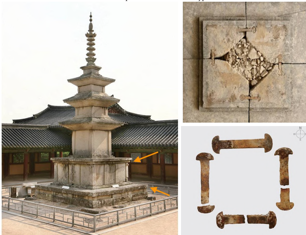
Fig. 16. Left: Three-story stone pagoda (“Seokgatap”), ca. 751, Bulguk-sa temple, Gyeongju (arrows point to clamp locations); Right top: Installation condition of clamps on the four stone-block assembly for the cover-stone of the upper-tier base; Right bottom: four extracted iron clamps of half-circle head type.
