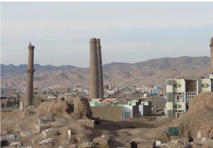
Fig. 23. New construction at north edge of Kuhandiz cemetery.
