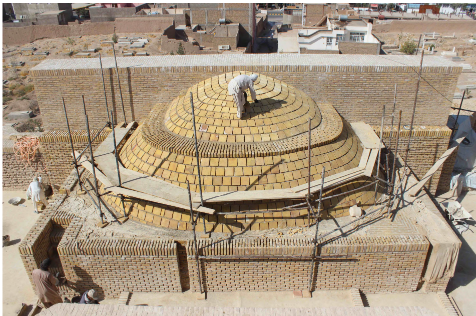
Fig. 11. Brick paving over reconstructed west iwān .
