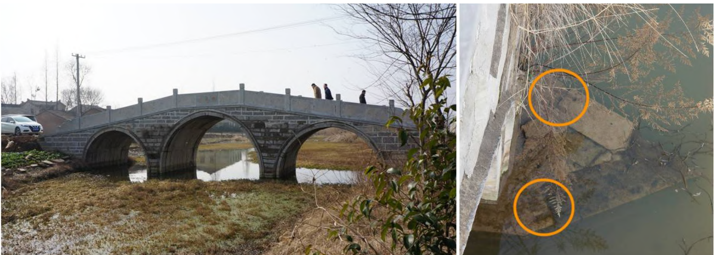
Fig. 13. Left: Yicheng Bridge; Right: Pier-stones with dumbbell-type clamps with circular head, Gourong City, Jiangsu. The pier-stones date from the Southern Dynasties (420–589), but the bridge is mostly late Qing reconstruction.
