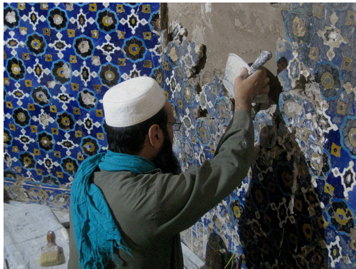
Fig. 19. Pouring gypsum plaster behind unstable mosaic faience.
