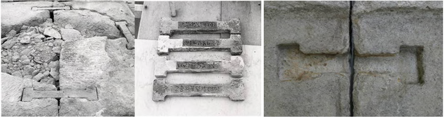
Fig. 14b. Left: Installation condition of four clamps on a four stone-block assembly; Center: four extracted clamps from the second level of the eastern pagoda; Right: Clamp-groove (square-head type) from topmost roof-stone of the western pagoda.
