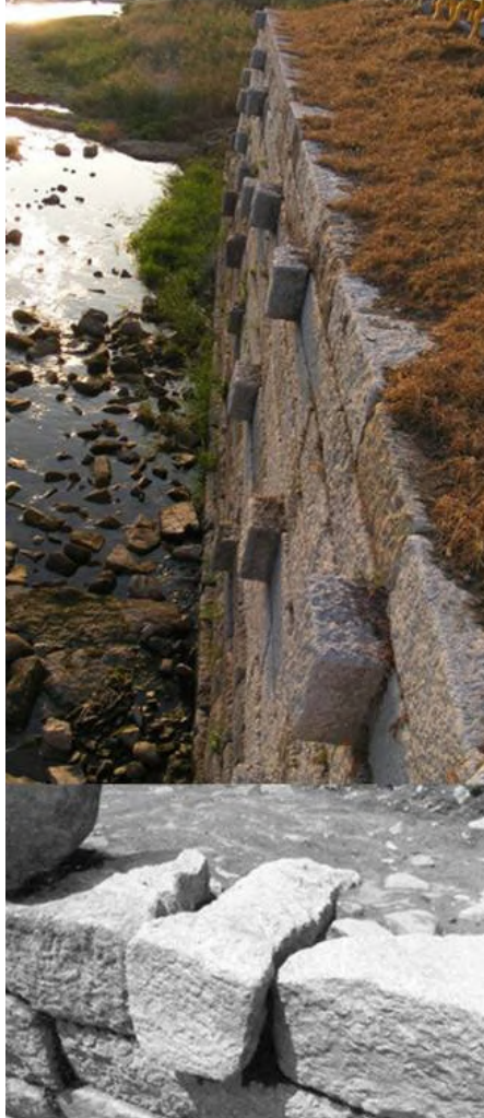
Fig. 18. Left top: One of the piers of the Woljeong-gyo Bridge, completed in 760, Gyeongju; Left bottom: Example of a half-circle head type clamp-groove on a pier-stone. Right: Reconstructed Woljeong-gyo at present. Center top: Stone-rivets on the north-side abutment wall; Center bottom: a detail of one stone-rivet.
