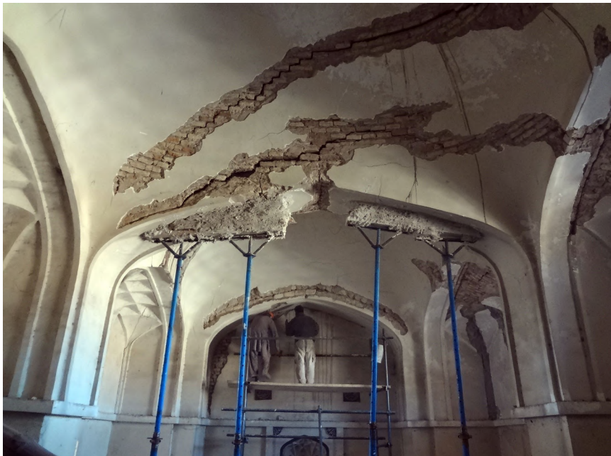
Fig. 13. Interior of mosque prior to reconstruction.
